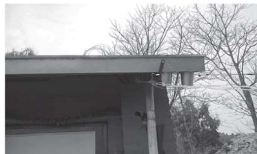
Gutter for Rain Water Harvesting
